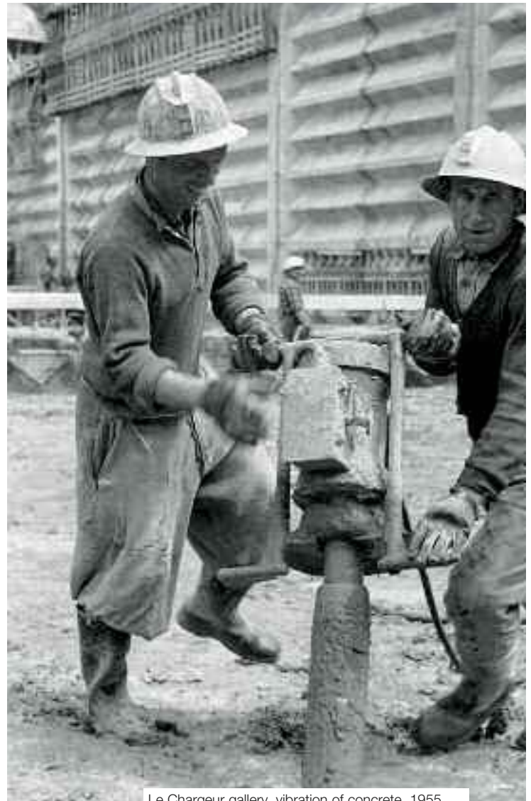
Le Chargeur gallery, vibration of concrete, 1955
