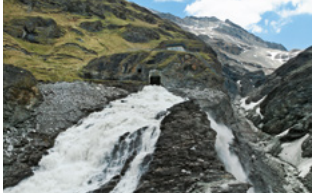
Inlet of the collector in the Lac des Dix in Cheillon
