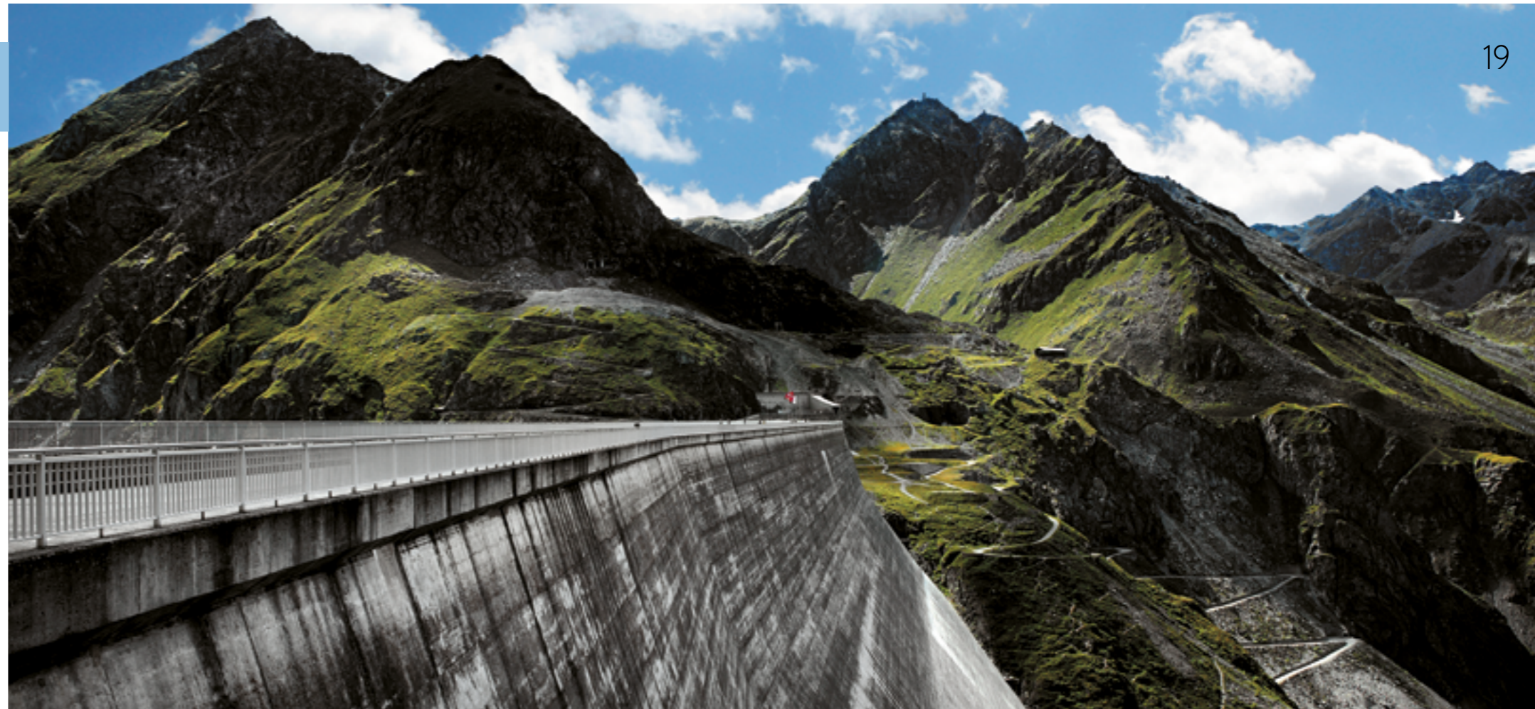
Walk around the top of the dam
