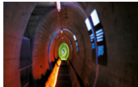
Tour inside the wall of the dam
