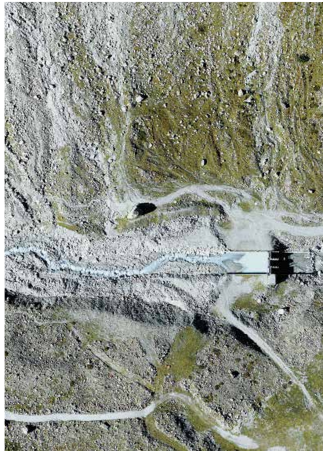
Lower Bertol water intake
