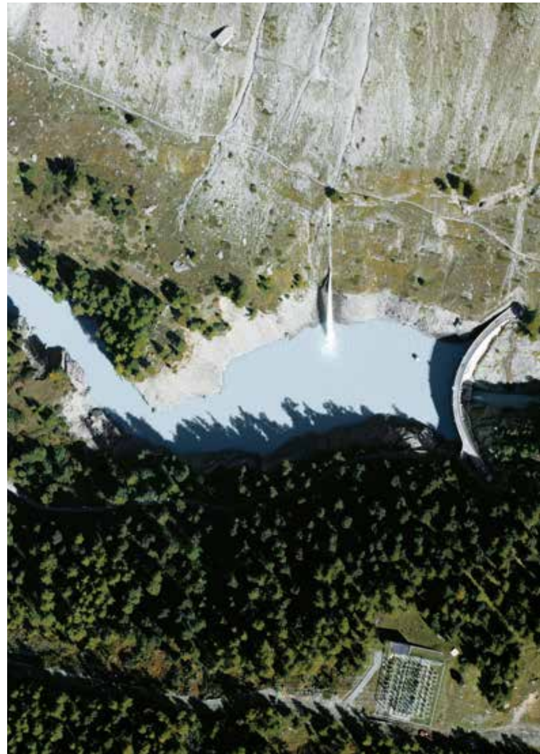
Z'Mutt afterbay reservoir at the foot of the Matterhorn
