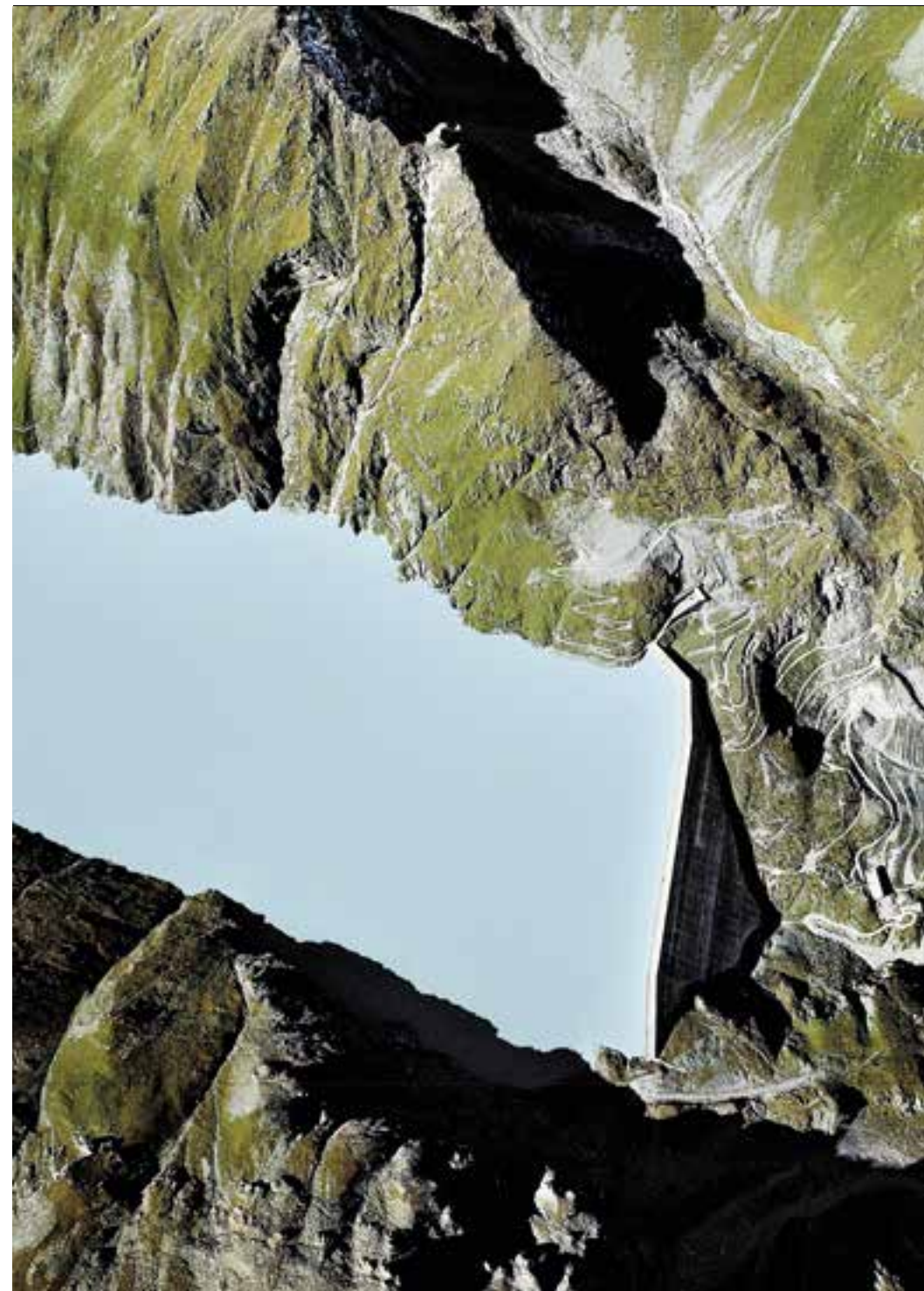
The Grande Dixence dam, the keystone of the hydroelectric complex
